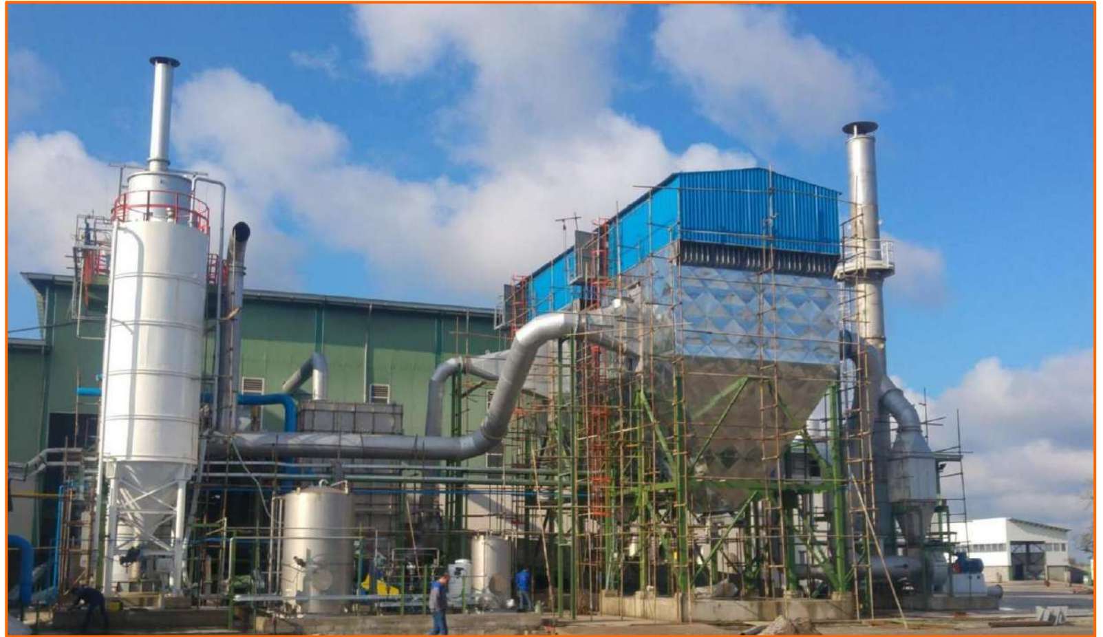
From left to right: Post-combustion chamber, Lime silo, baghouse filter and stack
