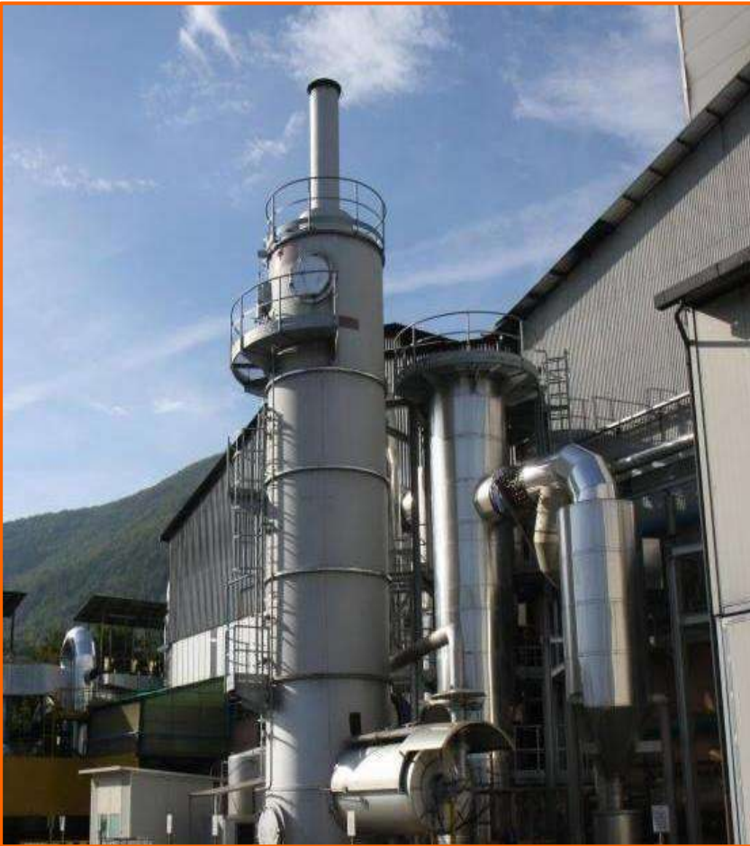
From left to right: Post-combustion chamber, Lime silo, baghouse filter and stack
