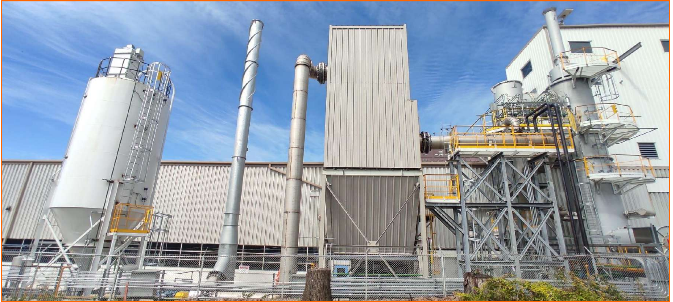
From left to right: Lime silo, Baghouse filter, post-combustion chamber
